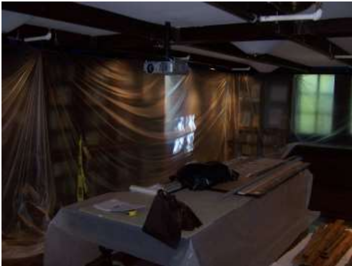
Photo #3: Workspace prepared
