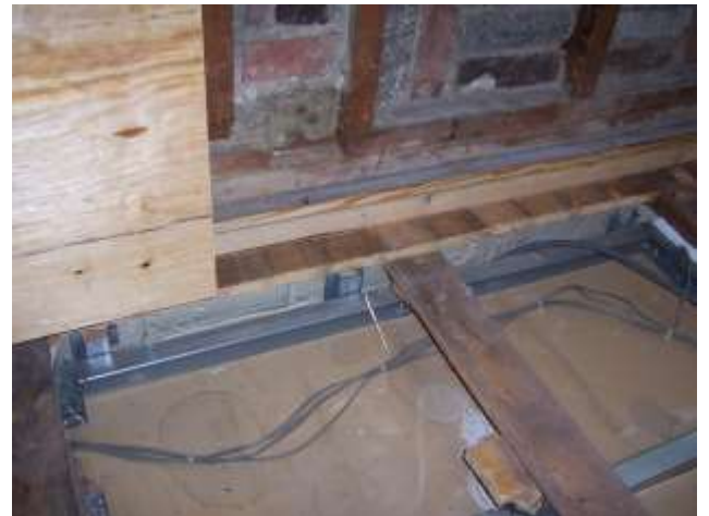
Photo #4: Floor strengthened for new lift installation
