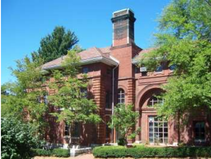
Photo #1: Building exterior
