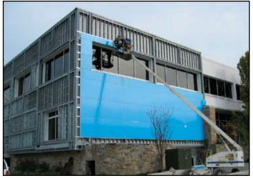
Welded Steel tube system has been installed and supported at the base. Cold formed metal stud framing and new facade installation is in progress.
