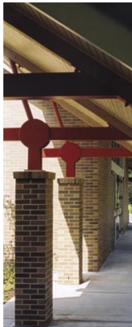
All photography for this article courtesy of Tellalian Associates Architects & Planners.
