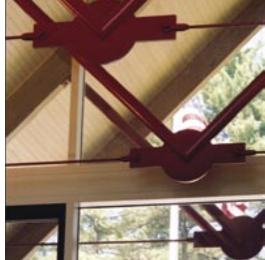
Circular gussets provide a clean, uniform appearance.
